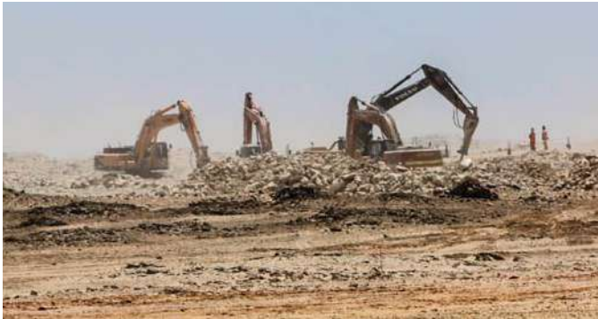
One of the sites overlooking the top of Ras Markaz where the oil storage terminal will be established
